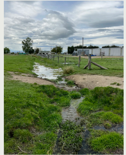
Culvert site in December 2021.
