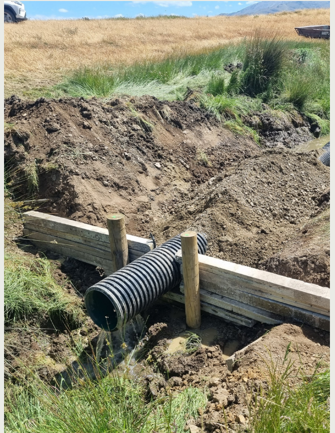
Wallington Road, installation.
