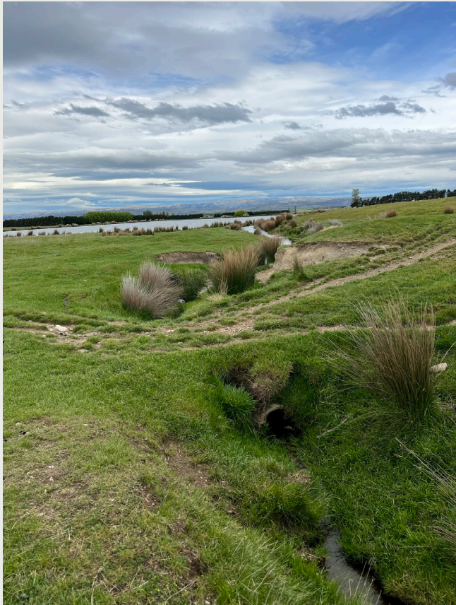
Wallington Road culvert and perched culvert prior to changes.
