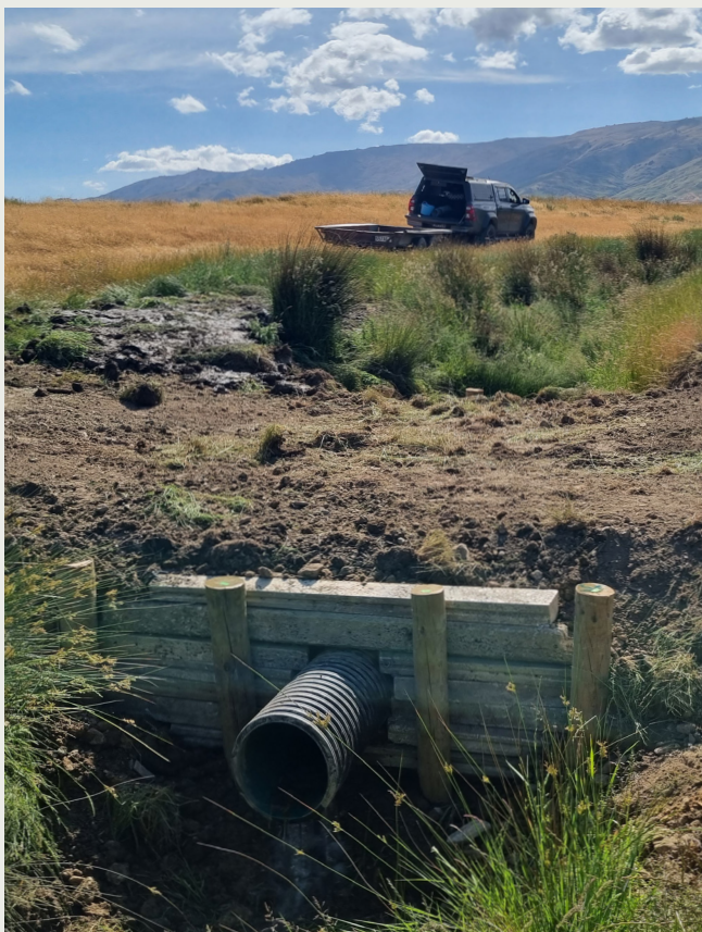
Wallington Road perched culvert prior to fence installation.
