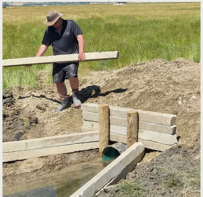
Installing the culvert sides.
