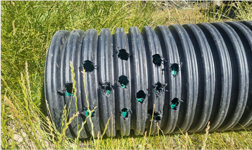
Holes drilled in the pipe to disperse water flow.
