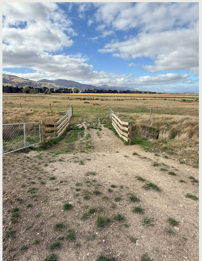
Wallington Road fenced culvert and creek March 2025.
