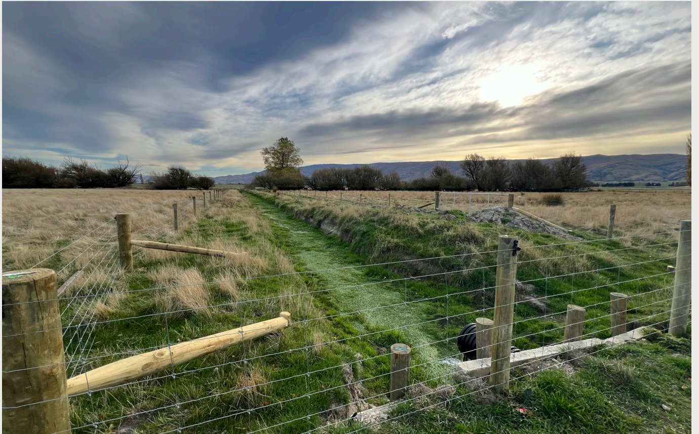
Downstream of culvert post works.
