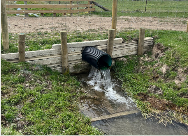
Completed Hepburn Road site.
