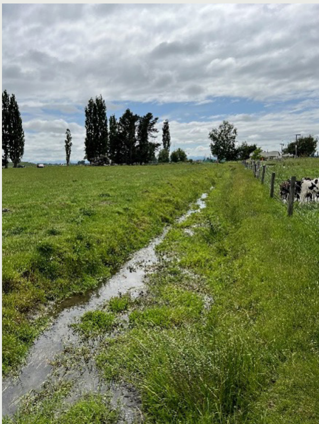
Upstream of proposed perched culvert prior to works.
